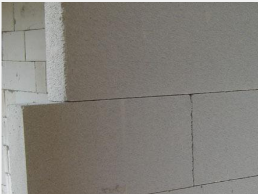
SeaRidge Uses Only High Quality Concrete Block
