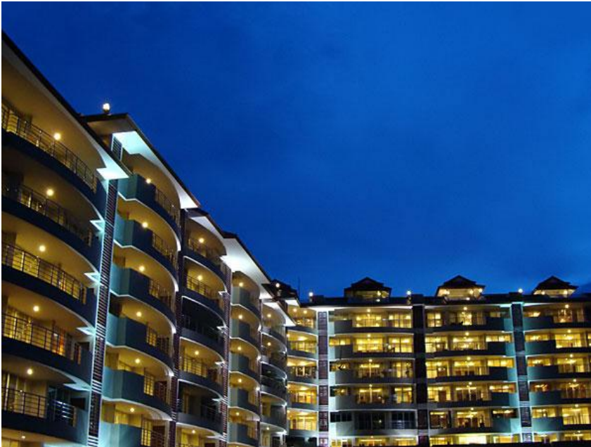
SeaRidge Condominium - Every Condo has Heavy Duty 100 Amp Electrical System
