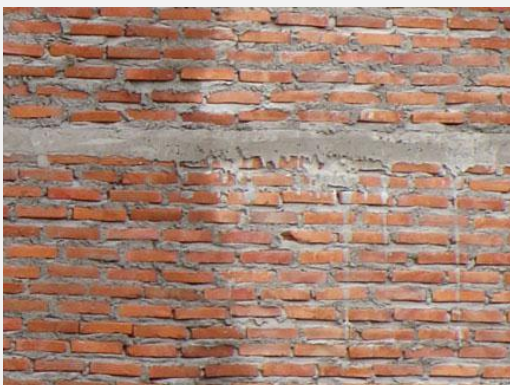
Low Quality Red Brick Construction
