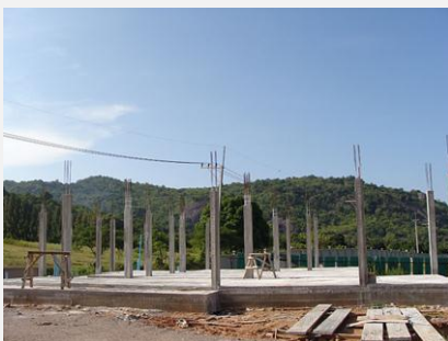
High Quality Home Foundation under Construction
