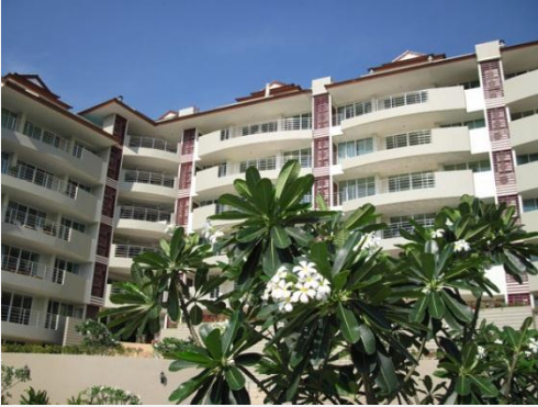
SeaRidge Condominium – Ready to Move in Now
