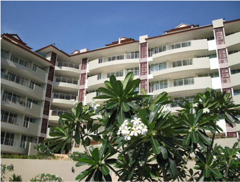
SeaRidge Condominium – Ready to Move in Now
